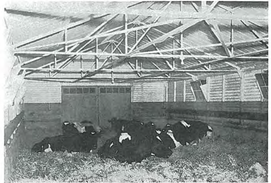
The cold, open, loose housing barn has temperatures from 8 to 10 degrees above outside temperature. The deep manure pack has a temperature of around 90° F. Comfort for the animals at these low temperatures seems to be adequate. Consider the bedded area as the bed room for cows to lie down. It should be bedded daily and no feeding or traffic lanes or holding of the animals on the bedded area should be permitted.
