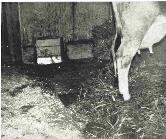
Figure 3. The outlet opening of the automatic barn cleaner may serve as the source of cold draft on udders of stanchioned cows.
