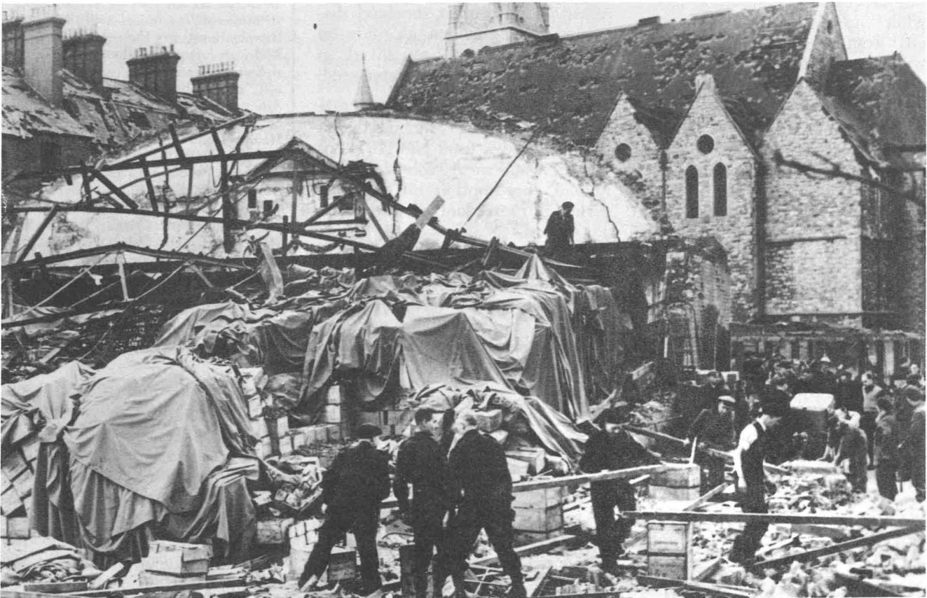
An example of successful British food salvage operations during World War II was the case of this building in which 650 tons of miscellaneous foodstuffs were stored. It was completely demolished in the bombing and everything inside seemed a total loss. Six weeks of careful work resulted in recovery of 636 tons of food.
