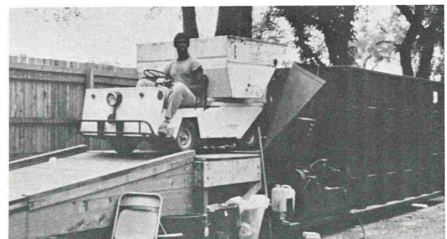
Figure 8. On-site solid waste compactor unit.
