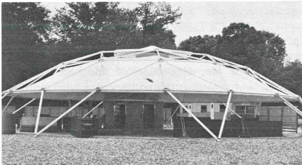
Figure 2. GSI Food Stand under construction.
