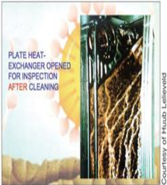
Figure 3. Example of a heat exchanger opened for inspection after CIP cleaning.
